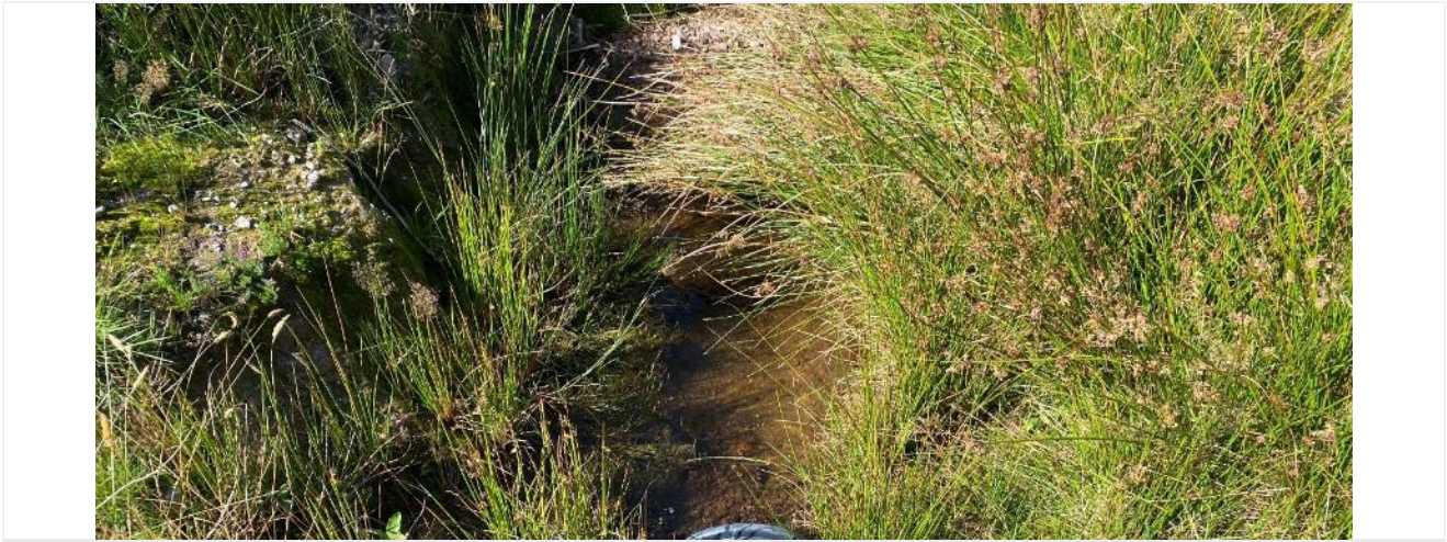
Image 9-13: Drainage Ditches FW4
