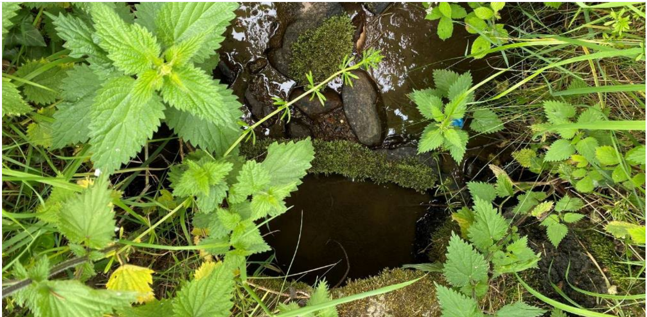
Image 9-17: Ballynaguilkee_Lower Crossing Point
